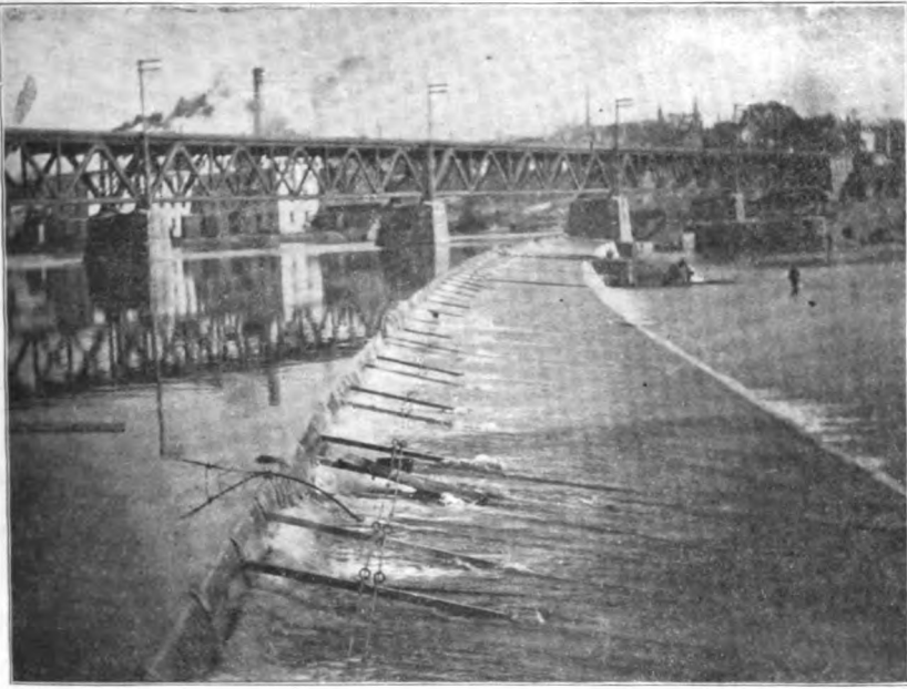
Fig. 375. — Flash Boards and Supports, Rockford Water Power Co.
