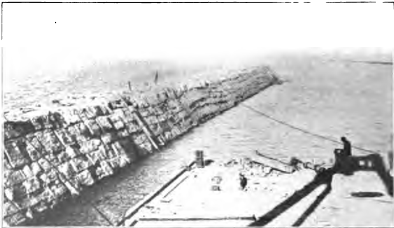
Fig. 33. Breakwater, Harbor of Buffalo, N. Y., with Facing and Top Stones Complete.
