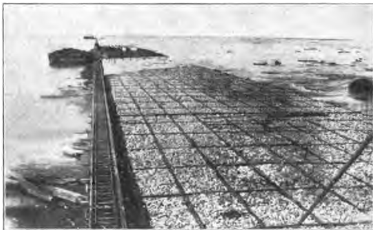
Fig. 12. One of the Huge Mattresses Used in Jetty Construction on the Mississippi River.
