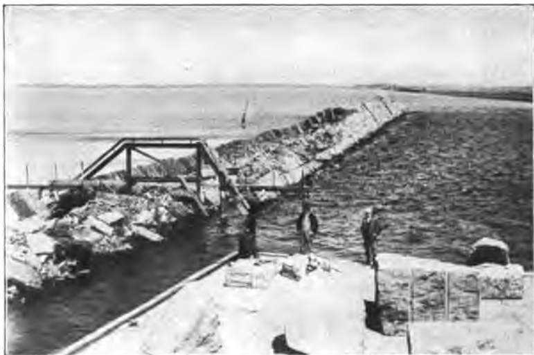
Fig. 31. Improvement of Harbor of Buffalo, New York. Showing method of constructing breakwater.
