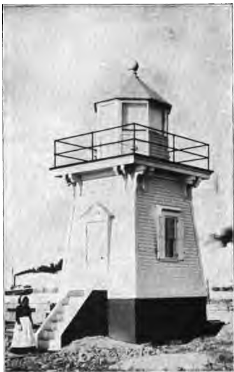
Fig. 47. Grassy Island Light Station, Detroit River. South Channel Range. Window beneath bal- cony faces south along range line.
