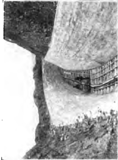
Fig. 145. Concrete-Lined Section of Truckee Canal, Nevada. Lining in rock cut, seventh section, looking downstream.
