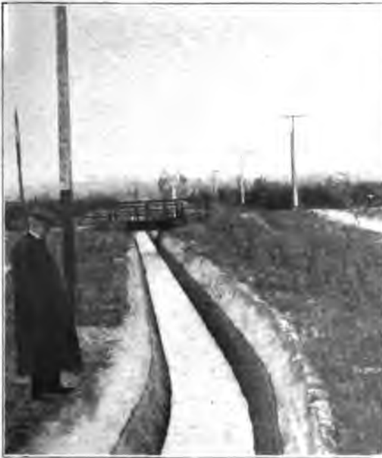
Fig. 149. Bear Valley Canal, Redlands, California. Boulder-lined and plastered. Courtesy of "Engineering News."
