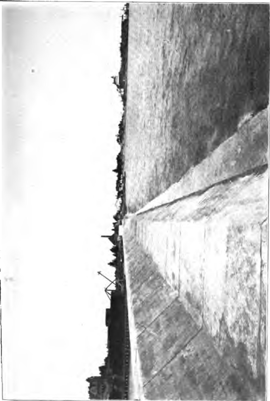
CONSTRUCTION OF CONCRETE SUPERSTRUCTURE TO BREAKWATER, MARQUETTE, MICH.
