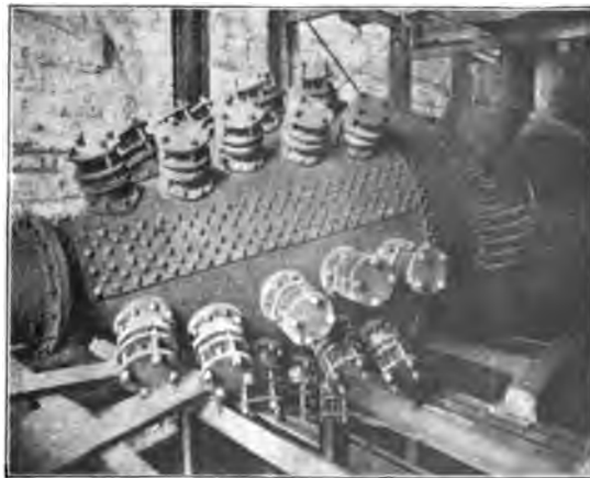
Fig. 168. Relief-Valves on End of Penstock.
