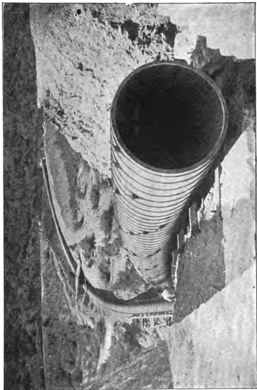
Fig. 138. Redwood Stavepipe (52-inch) Crossing Warm Springs Canyon, near Redlands, California. (Courtesy of U. S. Geological Survey.)
