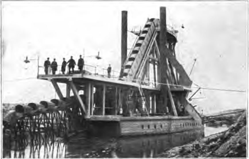
OLD-STYLE BUCKET DREDGE Cape Cod Canal.
