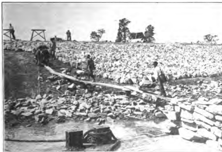
Fig. 10. Bank Protection on the Mississippi River. Placing the broken stone in position. Partially sunken mattress shown in foreground.
