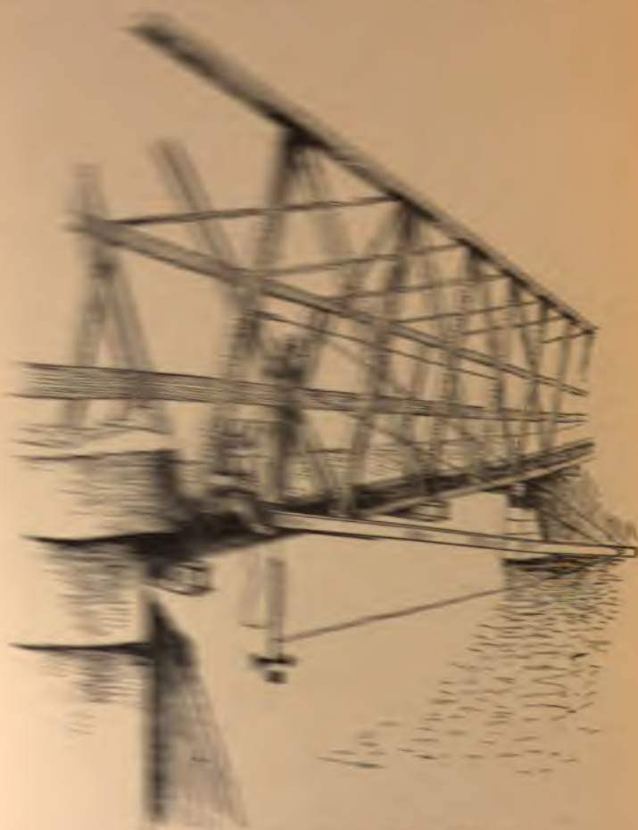
Fig. 1. Flume for Measuring Currents in a River.
