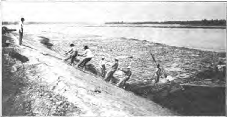
Fig. 11. Mooring a Mattress to the Bank of the Mississippi River.
