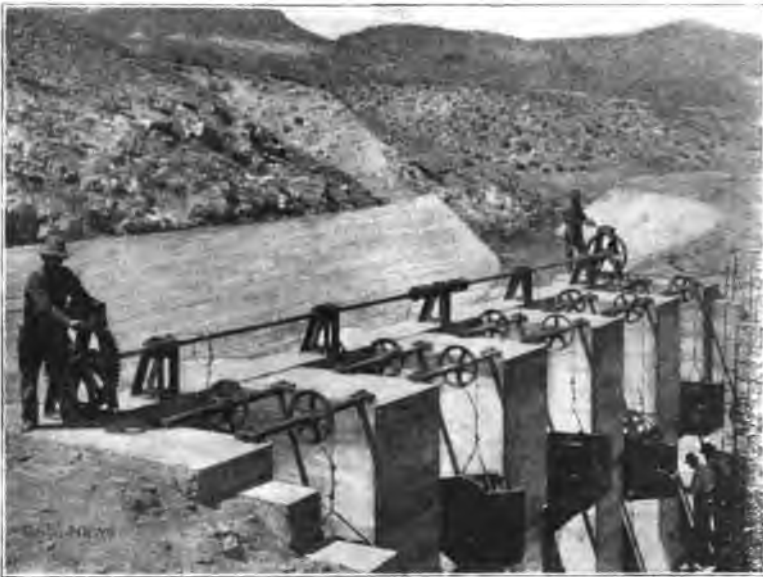
Fig. 160. Wasteway No. 1, Truckee Canal, Nevada. Showing mechanism for operating Taintor gates.
