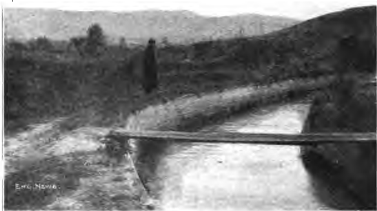
Fig. 147. Santa Ana Canal, California. Gravel concrete lining.
