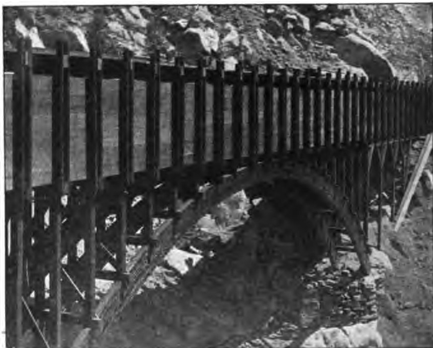
Fig. 154. Flume of Kern Valley Power Development Works, California. Courtesy of U. S. Geological Survey.
