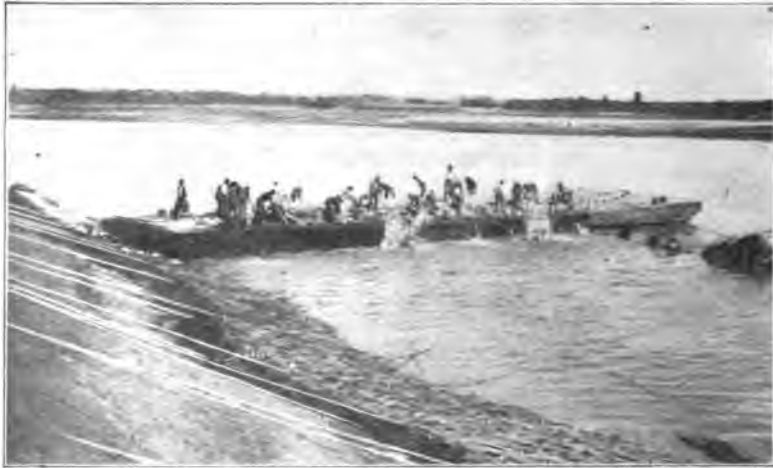
Fig. 13. Sinking a Mattress by Throwing Stones upon it from a Scow. The mattress is to serve as the foundation of a jetty for river-bank protection on the Mississippi.
