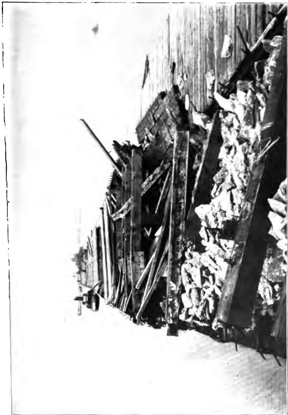
IMPROVING THE HARBOR OF CLEVELAND, OHIO Top of west breakwater after the destructive storm of November 10-11, 1918.
