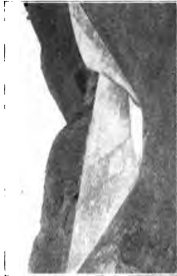
Fig. 146. Concrete-Lined Section of Truckee Canal, Nevada. Junction of earth and concrete-lined section, showing warped surface in latter.
