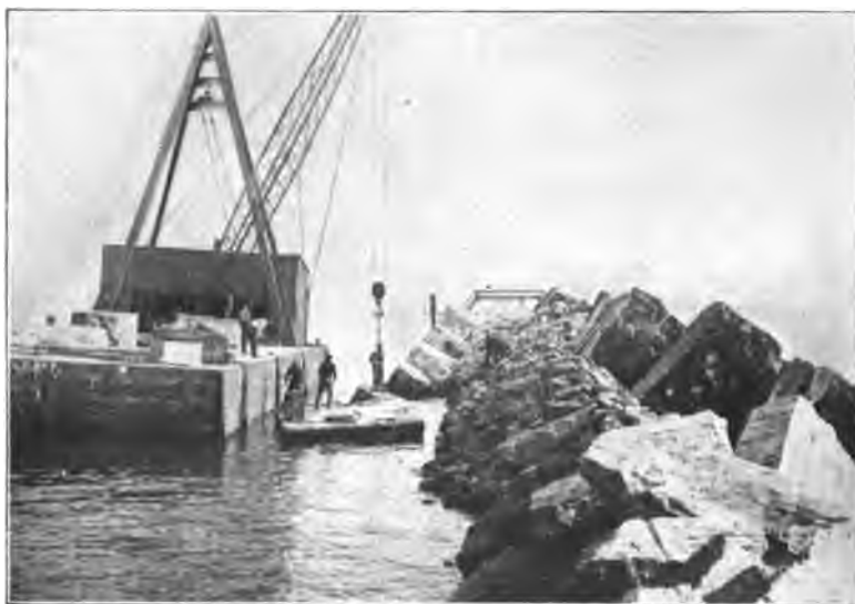
Fig. 32. Breakwater under Construction, Harbor of Buffalo, N. Y. Showing size of and method of placing facing stone.
