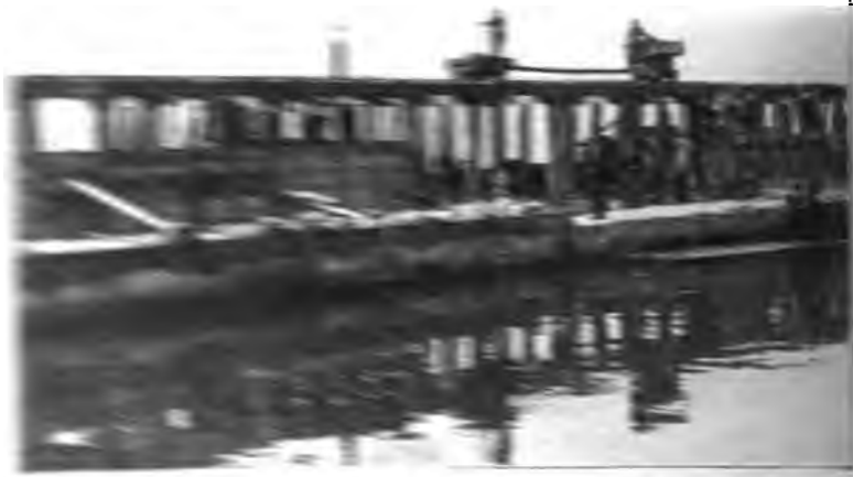
Fig. 1. Breakwater, Harbor of New York. Construction of breakwater, showing core of rubble masonry and concrete superstructure.
