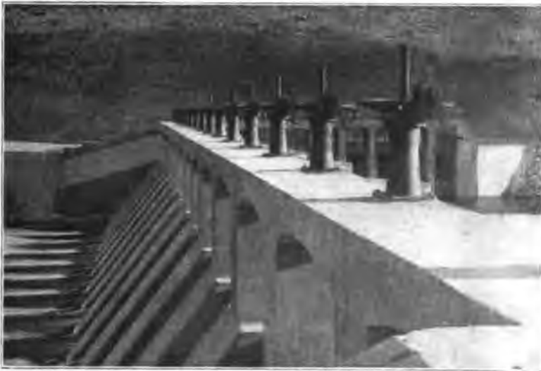
Fig. 161. Diversion Dam and Gates, Heading of Main Truckee Canal, Truckee-Carson Project, Nevada. View looking south along the dam, showing front face of dam; also the gate-operating mechanism.
