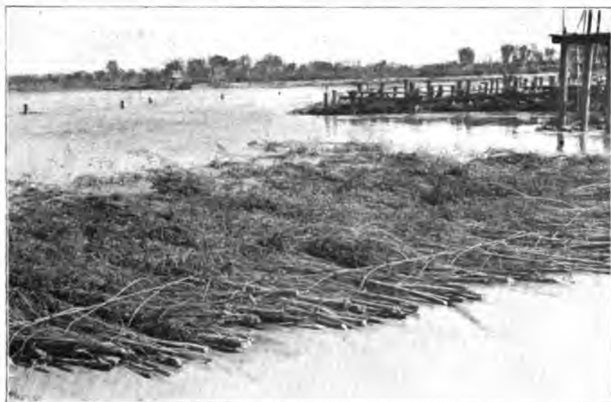
View Showing Brush Mat as Used in Constructing Dam.
