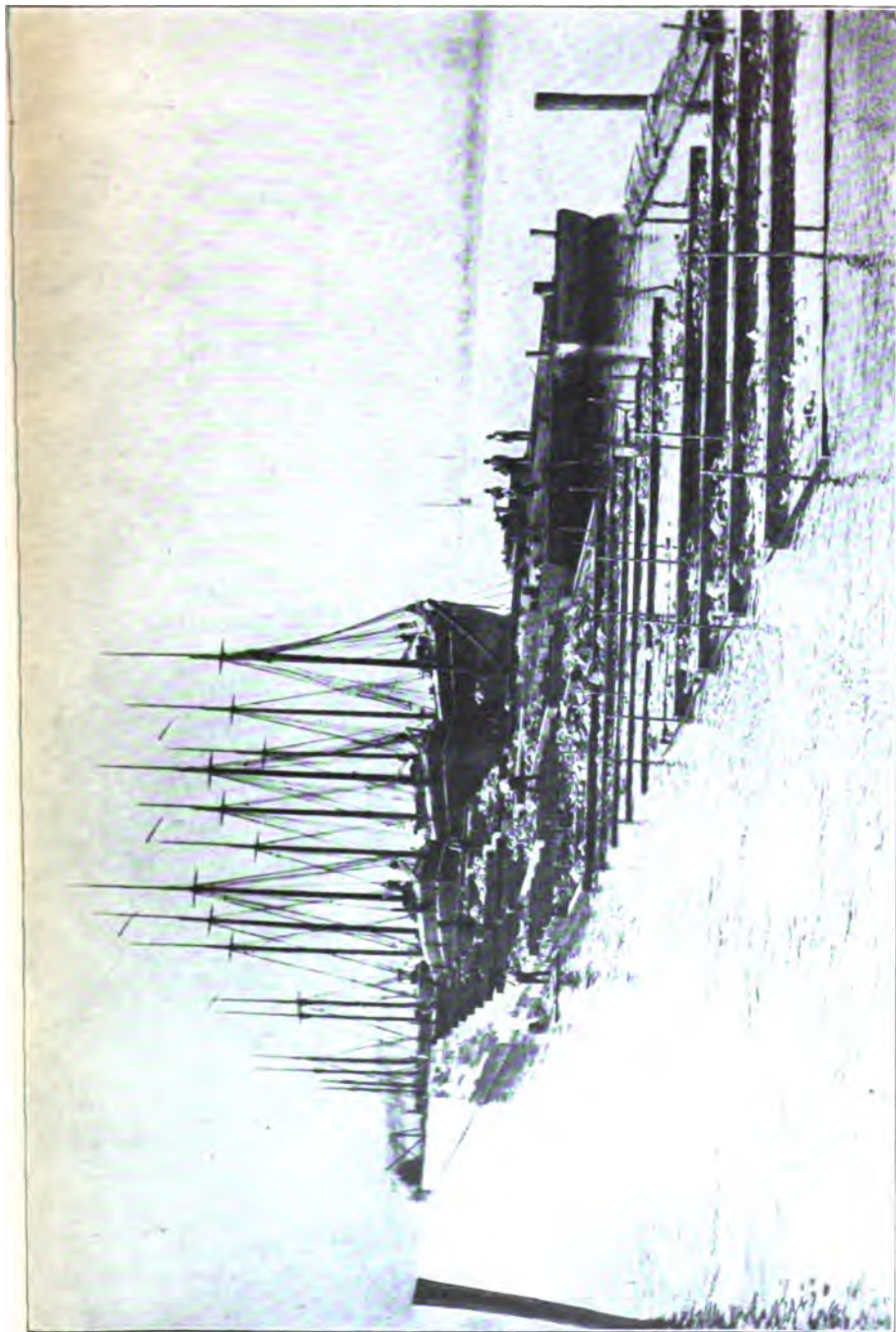
Fig. 27. Improvement of Harbor of Buffalo, New York. Breakwater under construction, showing timber cribwork extension at south end. The substructure cribs loaded with stone, are sunk in place, and the erection of the superstructure is shown under way.
