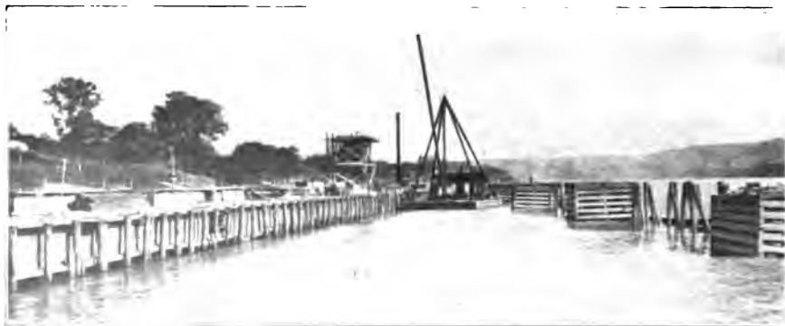
Cofferdam Used in Construction of the Dam at Fernbank.
