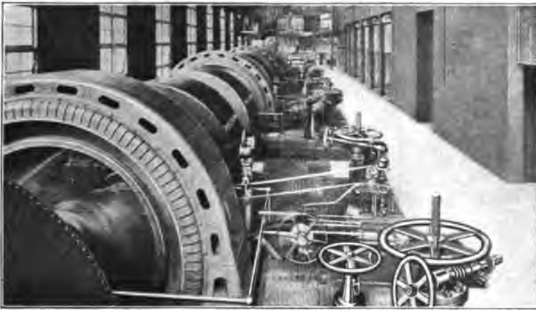
Fig. 46. Interior of Power House of Puget Sound Power Company, Electron, Wash. Four wheel units aggregating 30,000 h.p. in this station; of the "double-overhung" type, coupled to 3,500 k.w. 235 r.p.m. generators. Each unit has an overload capacity of 7,000 h.p.
