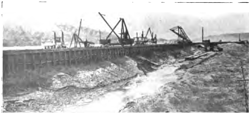
Main Guide-Wall of Fernbank Dam under Construction.
