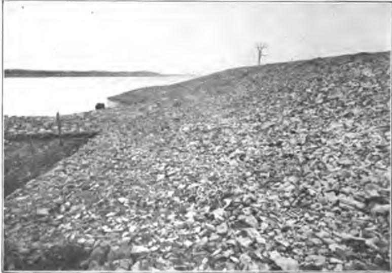
Fig. 9. Bank of Mississippi River Covered with Rubble to Protect it against Erosion.
