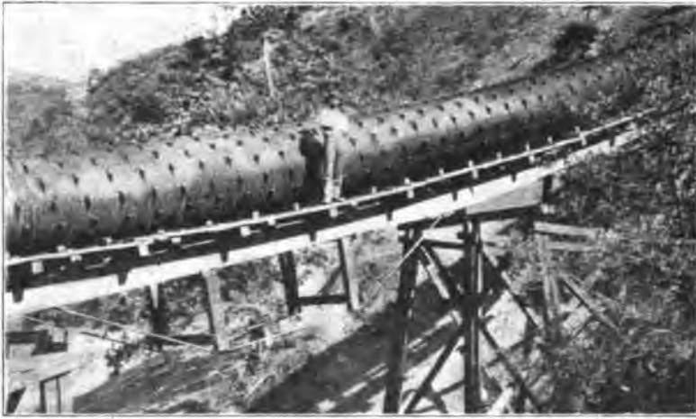
Fig. 137. . Redwood Stavepipe under 160 Feet Head. Santa Ana Canal, California.
