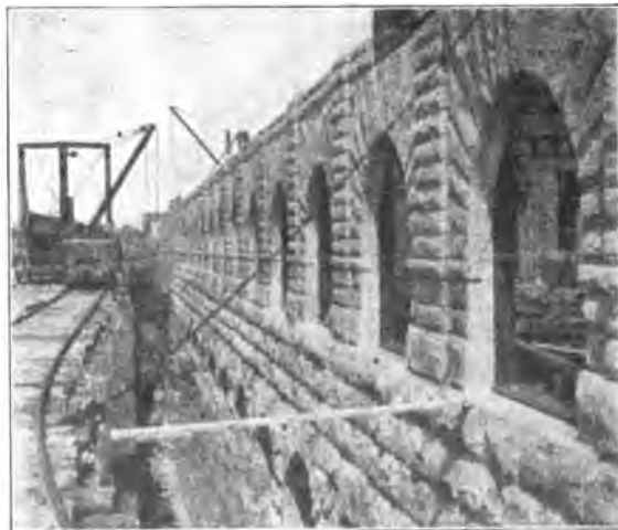
Fig. 174. Arched Entrances to Inner Forebay of Power-House No. 2, Niagara Falls Power Company. Entrances in lower wall, submerged when in operation.
