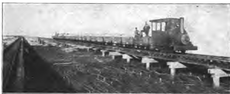
Fig. 14. Building a Mattress from a Trestle where Water was Too Shallow to Allow of Bringing in a Mattress which had been Built on the Regular Mattress Building Ways.
