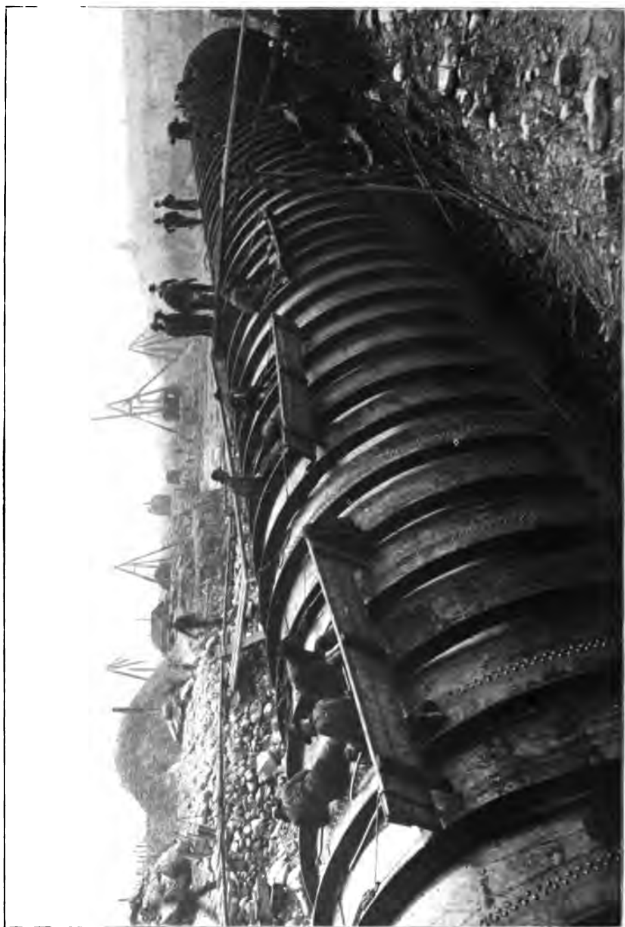
RIVETING DECK BEAMS ON THE STEEL FLUME OF THE ONTARIO POWER COMPANY, NIAGARA FALLS, ONT. Flume 18 feet in diameter, afterwards inclosed in a sheathing of concrete.
